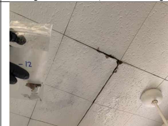
Photo of HA number 4, Non-ACM White 12"x12" Ceiling Tile (No Mastic), within Ceiling of Crafts Room and Office
