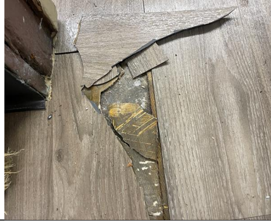
Photo of HA number 6, Non-ACM - 2'x4' ceramic floor tile (under the VFT)
