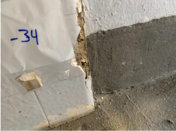
Photo of HA number 11, Non-ACM White 6"x6" Wall Tile, within Select Walls in Bathrooms
