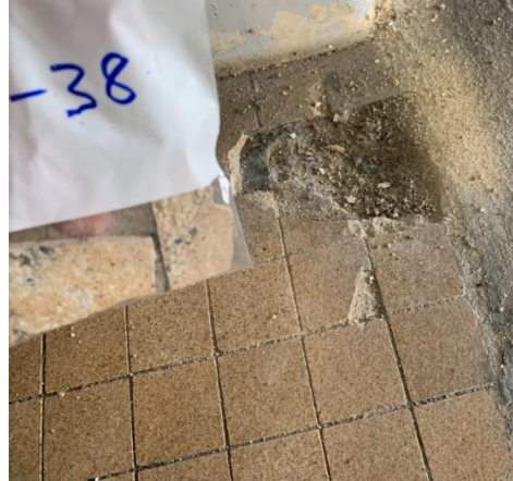
Photo of HA number 12, Non-ACM Brown Floor Tile (Bathrooms), within Select Floors in Bathrooms
