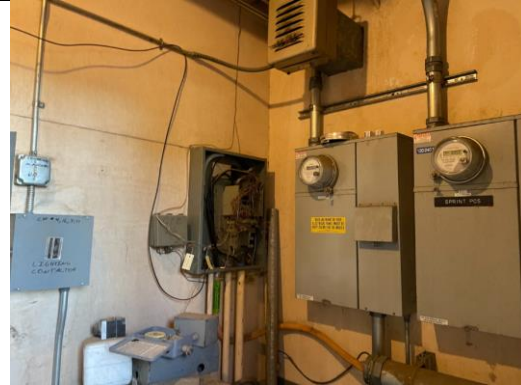
Photo of HA number 13, Non-ACM Gray Plaster Wall within the Electrical Room
